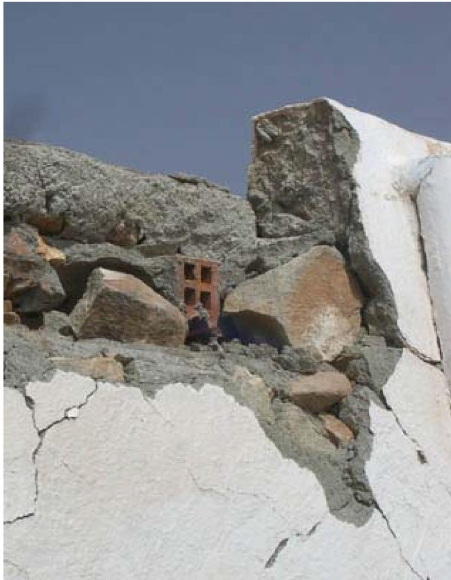
2.3.1 In today's traditional construction, small beams are cast using bricks as formwork, incorporating a single rebar for small spans in housing. Although hardly a moment resistant connection, there are shades of increased performance by the semi-diaphragm action resulting from this construction detail.
