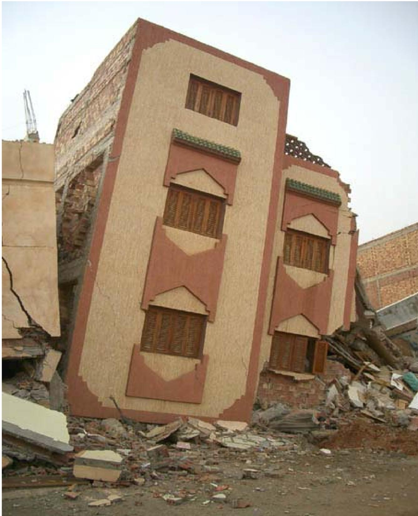
7.1.1 The building from the front, with ground floor collapse. (*grade 5 Vulnerability C*)
