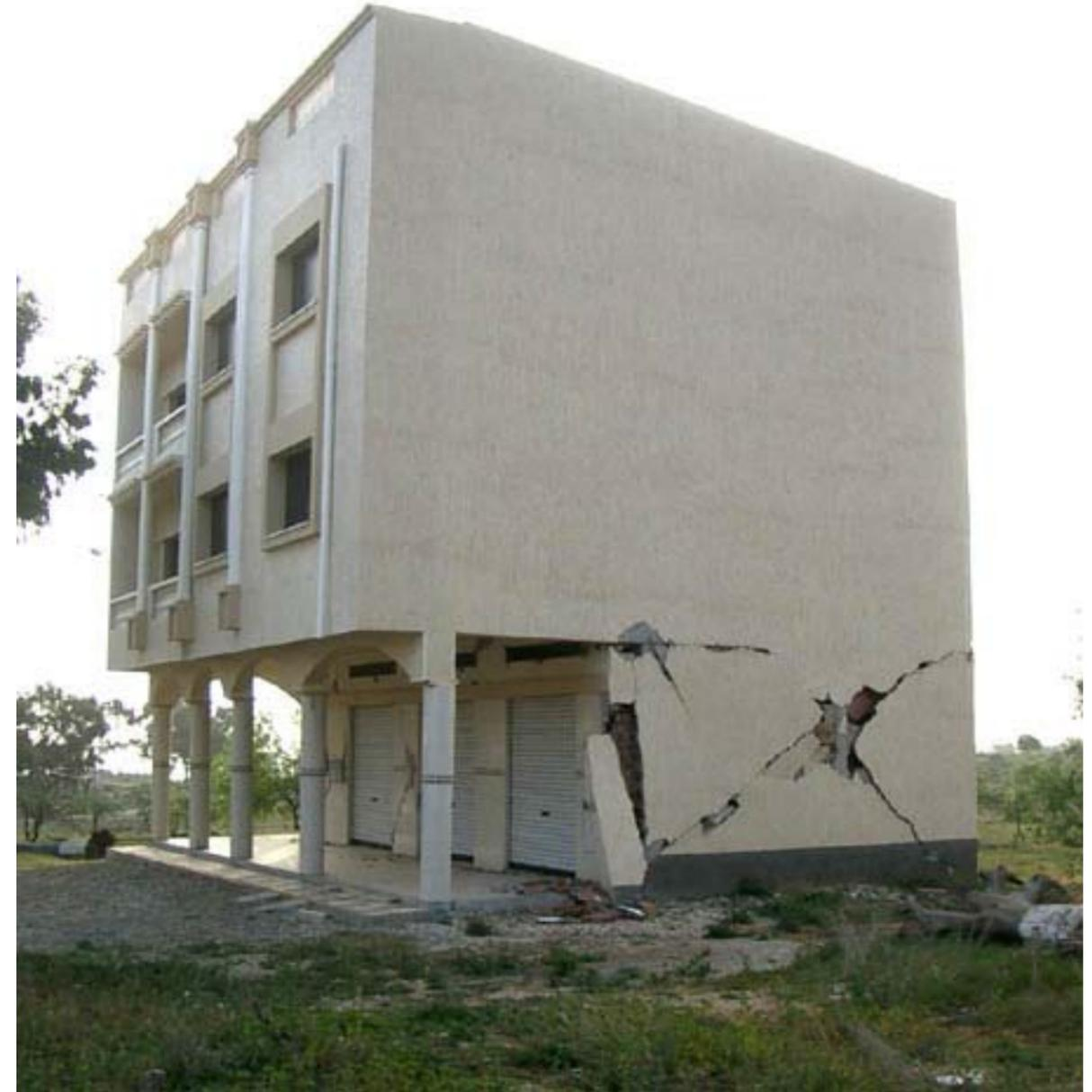
4.8.1 In an idealised situation the structural response to lateral loading is as the top model. However to perform as expected, the structure must be the stiffest element and the non-structural partitions must not compromise the ability for the structure to perform.
