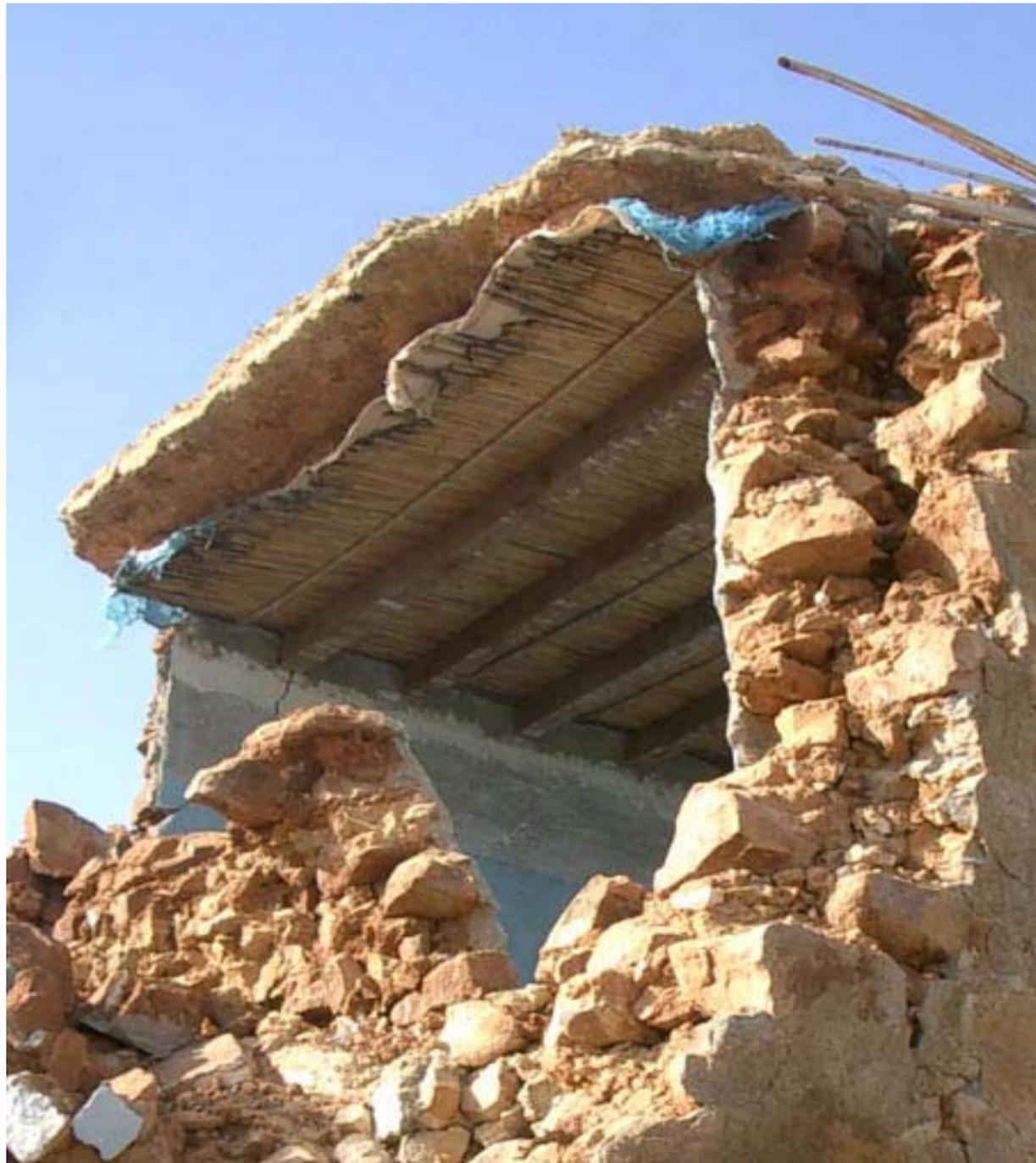
2.2.1 Traditional roof construction with a mortar screed laid over canes and wooden joists, a weak diaphragm action.
