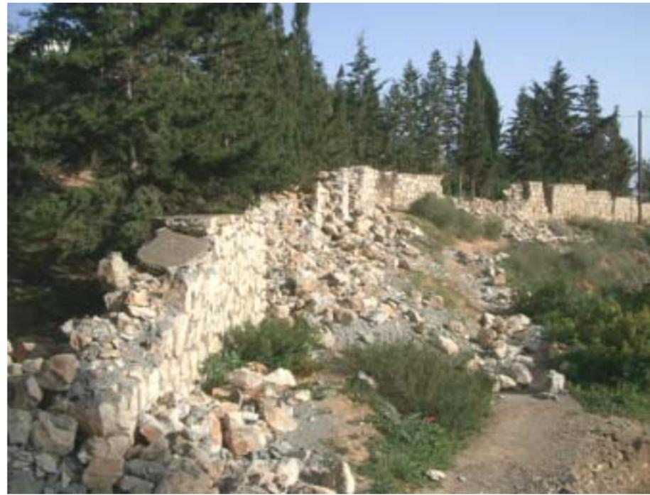
3.1.5 Brittle failure of masonry wall - Ajdir
