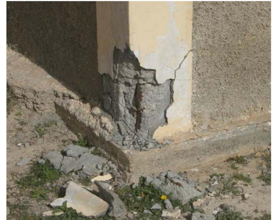
9.6.3 Spalling of concrete; the beginning of a plastic hinge.
