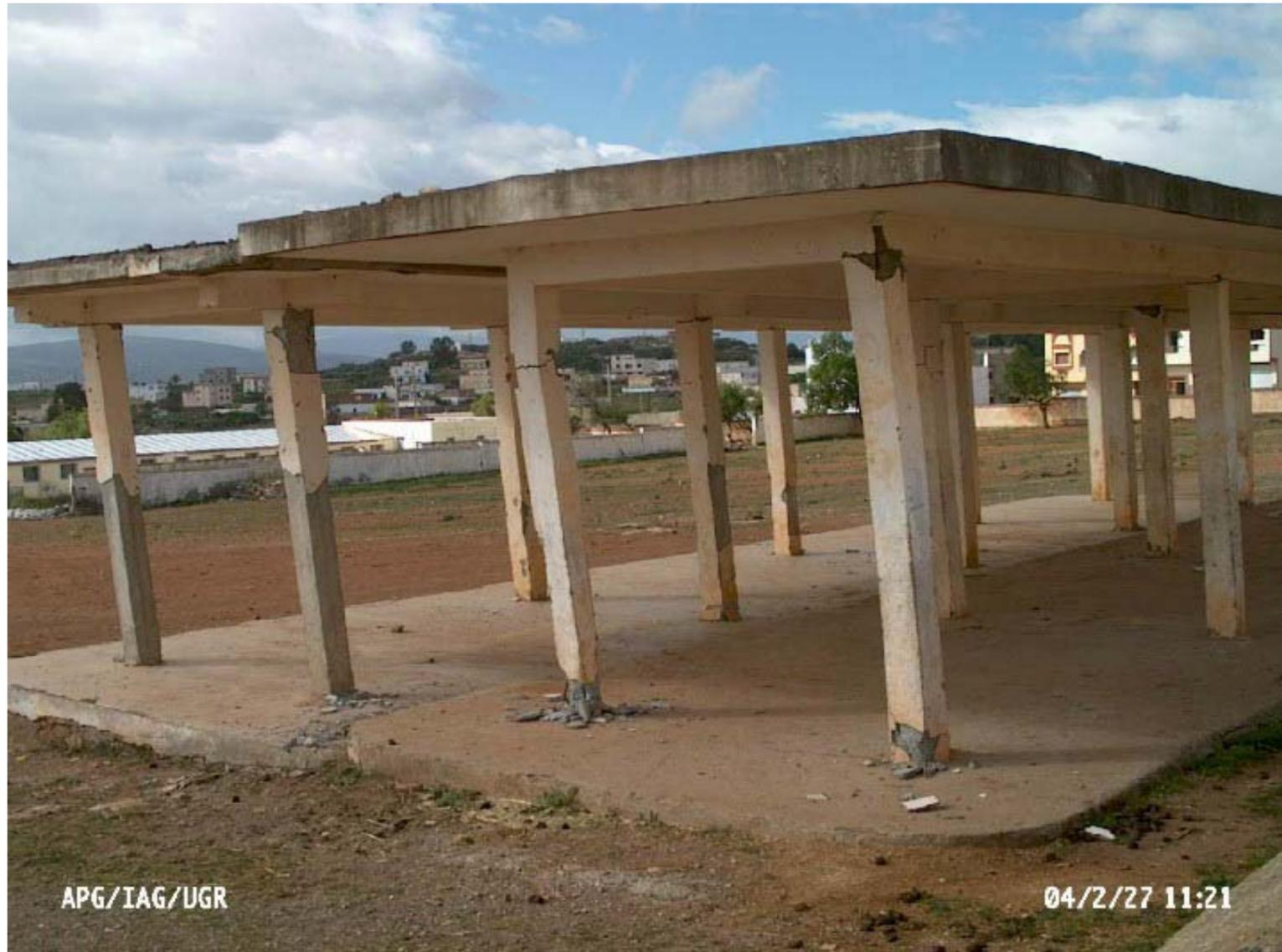
4.1.b.1 Plastic hinges at base and top connections. This is a non-ductile brittle RC frame in Izemurenne. Photograph courtesy of Mercedes Feriche
