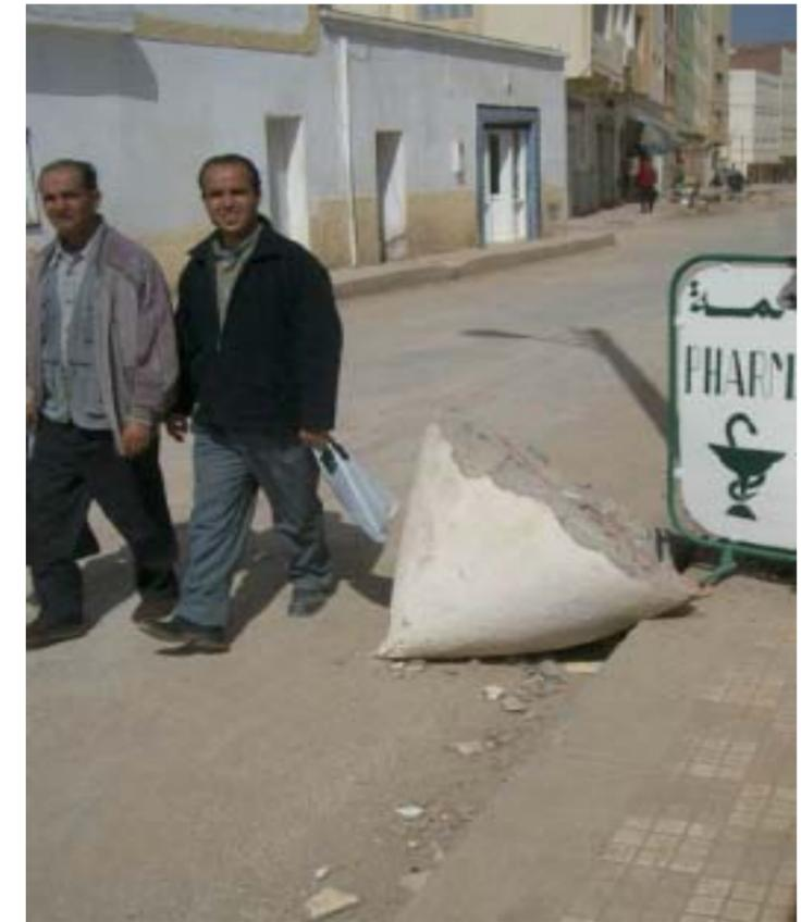
9.5.1 Here the lantern was knocked over (1) striking the entrance area (2) finally rolling over the road. (3) (grade 2 Vulnerability C – some may argue grade 3 'chimneys break at roof level')
