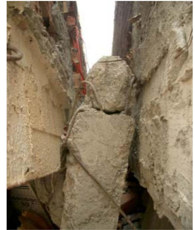
7.2.3 Column head detail. Note plasticated non-corruugated steel and small column section.
