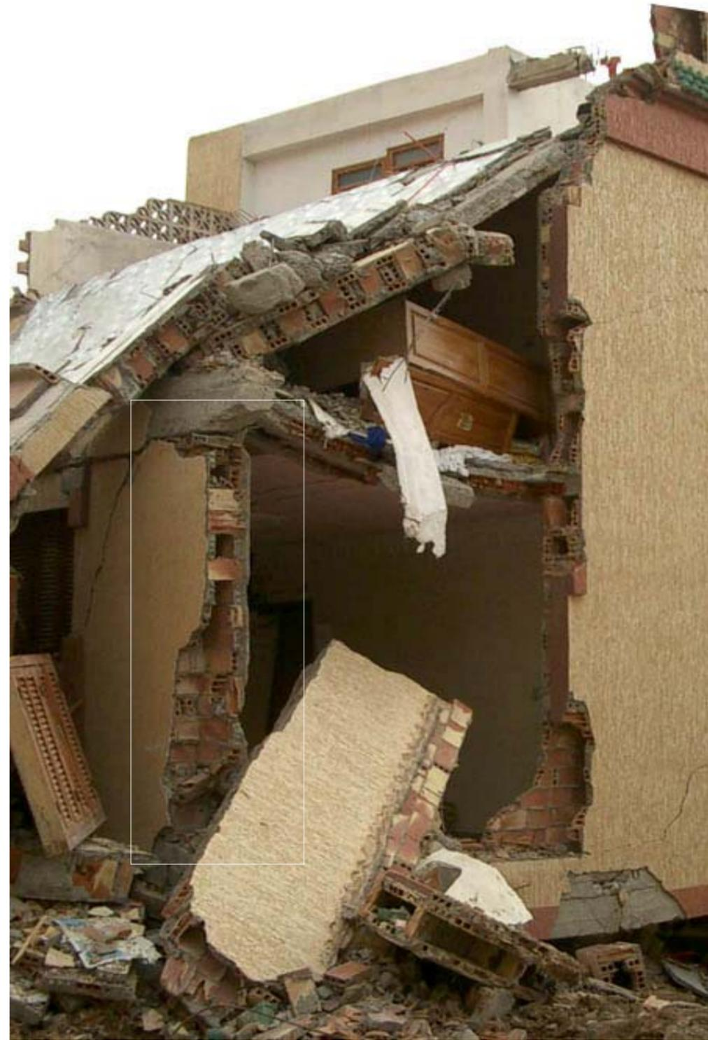
4.2.2 A collapsed RC building in Al-Hoceima showing external skin construction.
